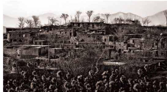
Figure 3 Villager residence building of Shuiyu Village in Luquan
